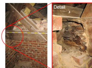
Figure 19: Heart rot damaged head in load-bearing joist at opened brick work
