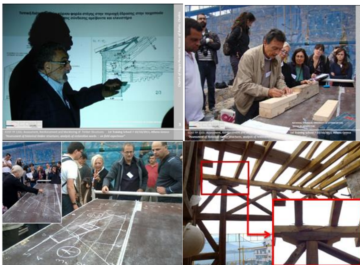
Figure 2: Historic timber buildings assessment: interpretation of survey drawing, on site design and sizing of repair timber to timber beam connection; implementation of the double scarf joint in a real structure.
