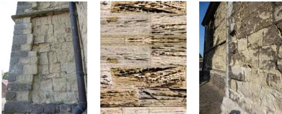
Figure 1: unfixing (left), loss of matter (centre) and cracking (right) [after 5]
