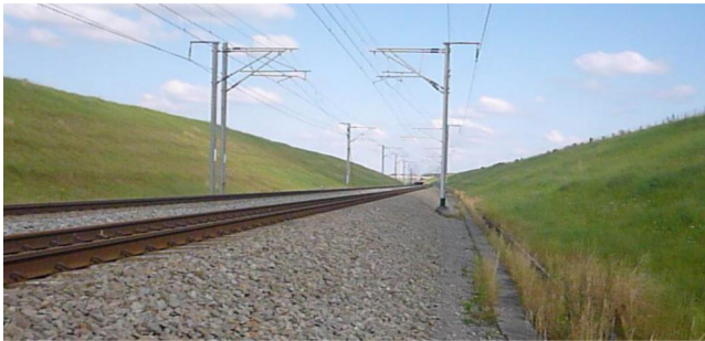
Fig. 7. Cutting track section.
