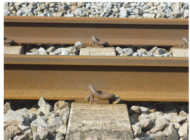
Fig. 3. Ballasted track configuration (all sites).
