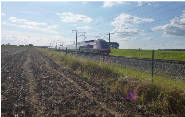
Fig. 1. At-grade track section.
