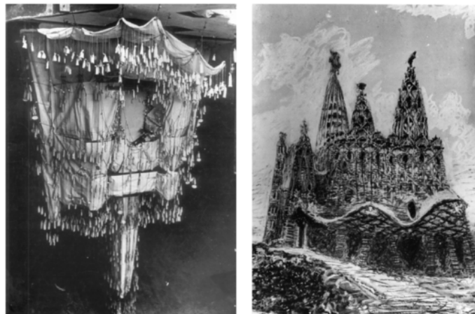
Figure 2.19: Gaudí's hanging model and resulting rendered form. Reproduced from (Maher & Burry, 2003).
