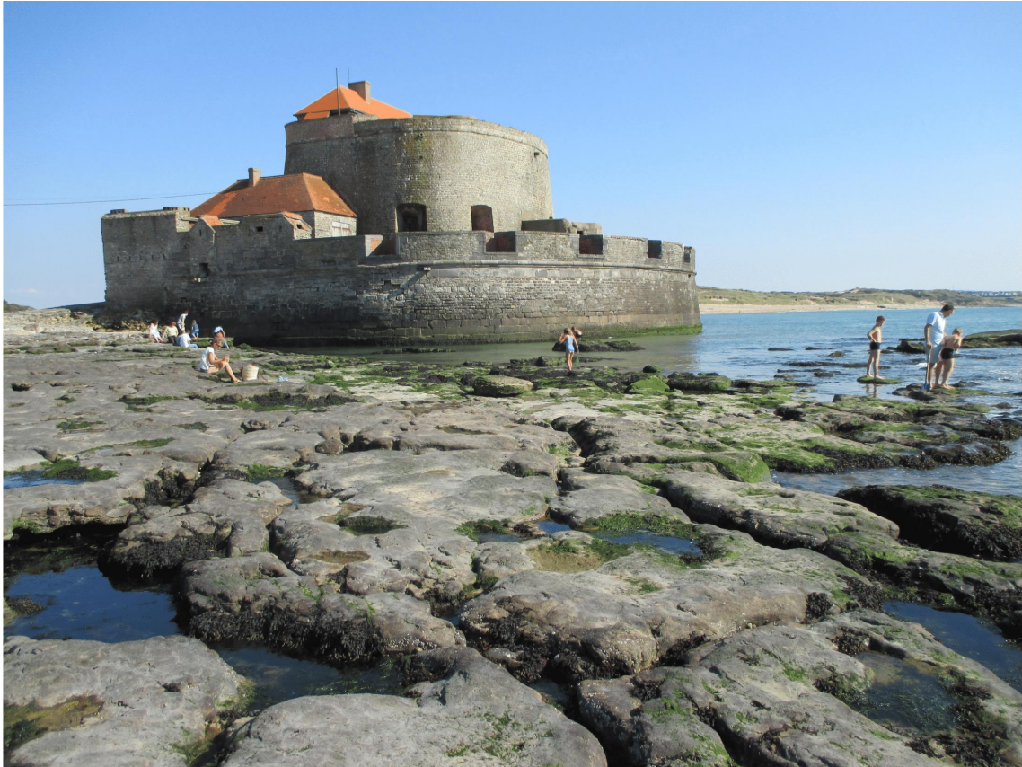
17th century Fort Mahon or Fort d'Ambleteuse standing on the Grès de la Crèche Formation and built with the same material (© R.Dreesen)
