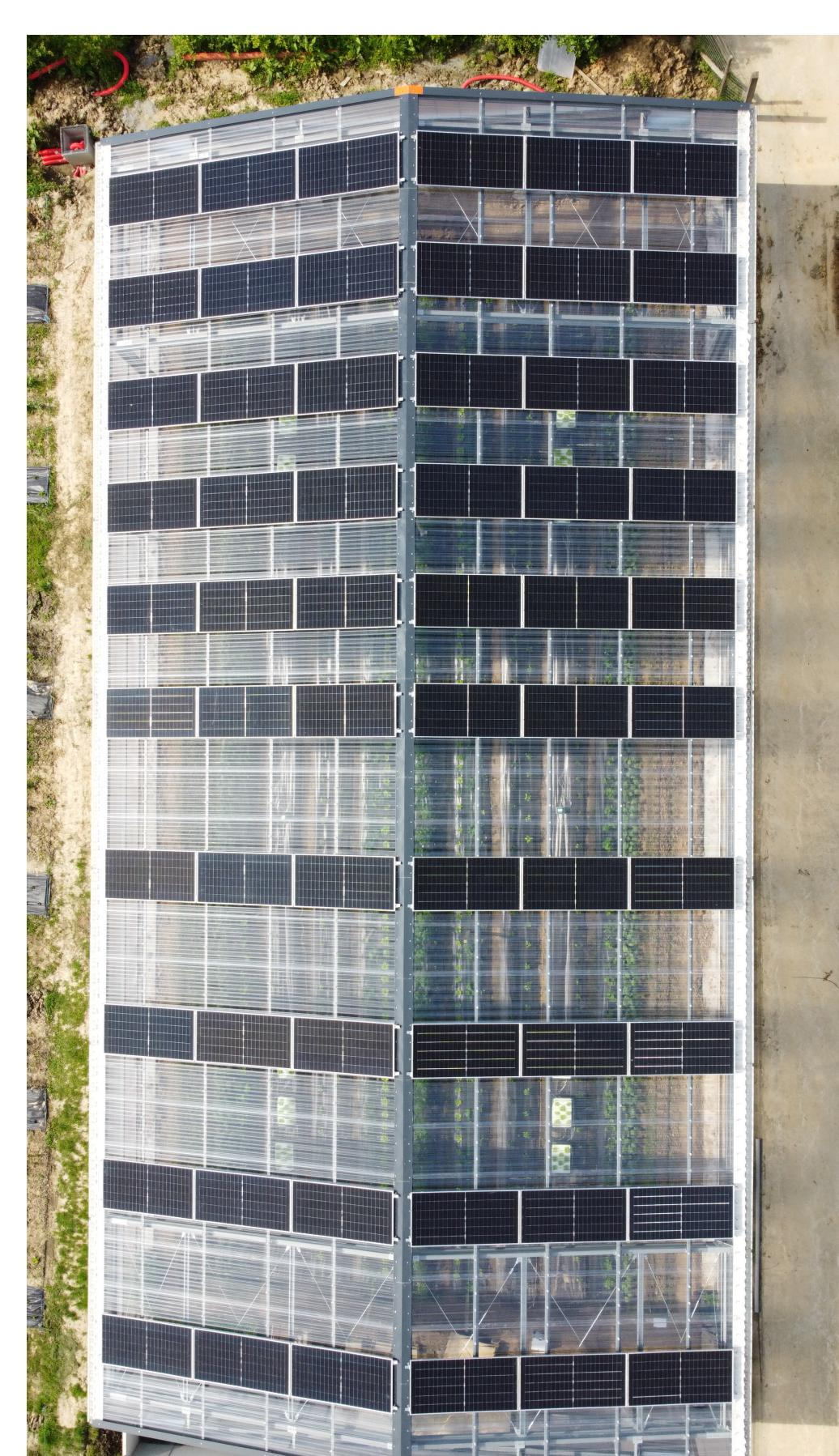
They serve as references to compare the crop growth and also to collect important data, used for the validation of the numerical model. The rooftops are covered with photovoltaic cells representing 50% or 30% coverage. The impact of the coverage on the crops is monitored on different growing beds. Several control means are considered to preserve a suitable climate for crop growth.
