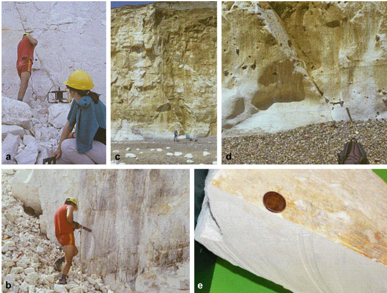
Fig. 2. Views of the fault planes. (a) Fault plane in the Harmignies quarry. The fault plane is roughly perpendicular to the quarry face. (b) Close-up view of a fault plane in the same quarry. (c) Normal faults in the Newhaven cliff. (d) Close-up view of the Newhaven sampling site. (e) Block showing striations on a fault plane in White Chalk. To the naked eye the chalk close to the contact seems to be unaffected by deformation.
